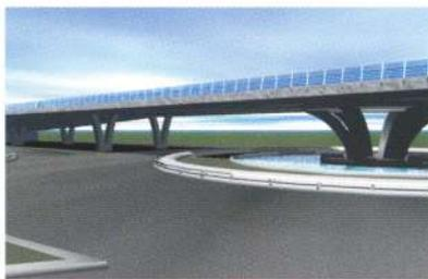
The viaduct proposed here features two continuous twin slabs placed side by side, in pre-compressed reinforced concrete, on 8 bays: 6 intermediate bays of 33 metres and 2 end bays of 24 metres, with a central "lily-shaped pier" with a span of 14.20 metres. The total length is 260.20 metres.
