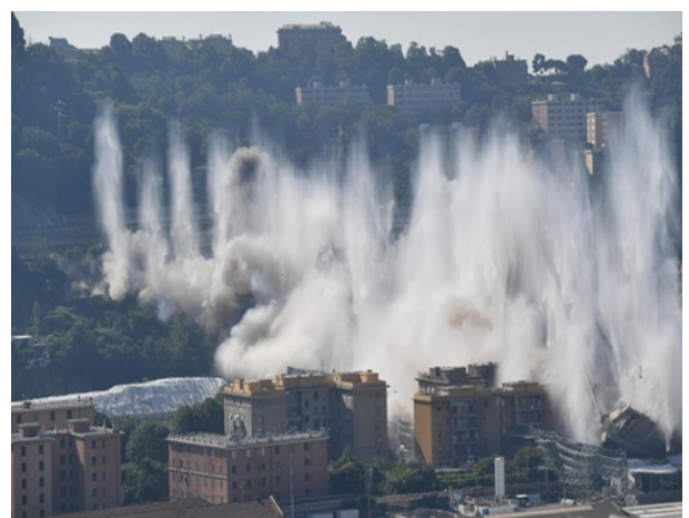
Figure 5- View by Sky TG24 of the whole demolition in June 28, 2019 of the Morandi Bridge using explosive microcharges to destroy all the structures including the repaired sound piles supporting the viaduct for more than 650 m (2,132 ft)
