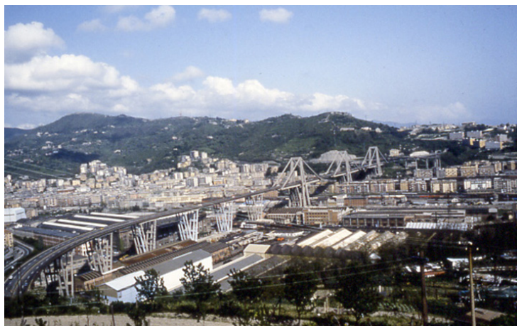
Figure 3- View of the numerous sound and crack-free white piles supporting the roadway of the Morandi Bridge repaired in 1982
